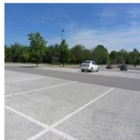
Figure 2. Parking Lot With Permeable Concrete. Permeable surfaces allow stormwater to pass through to the soil, decreasing runoff, improving water quality.
