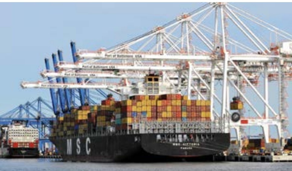
Baltimore's Seagirt Marine Terminal due to infrastructure investments can handle the new-Panamax container ships.
